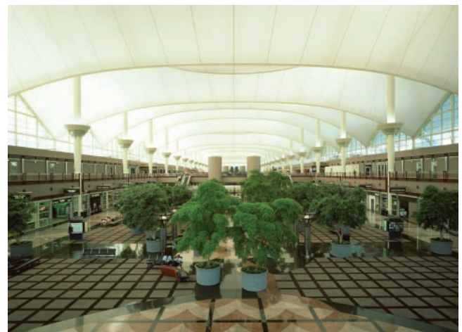
Figure 1: Daylighting at Denver International Airport Translucent roofing material and abundant windows at Denver International Airport provide natural daylighting.
